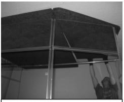
**12.** Lay STS trapezoids on either side of center lid section. Leave at least an inch over-hang in front. Make sure AX height extenders stay upright and perpendicular to floor.
