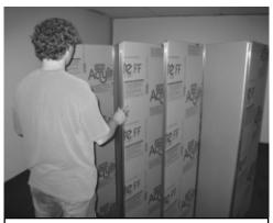
2. Stand up the main shield system in zig-zag formation, base channel on bottom.
