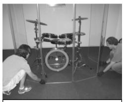
9. Use your fingers to lift the panels at bottom cable cut-outs to pull or push system into final position. End panels should be near parallel and symmetrical on either side of kit, 6 to 7 feet apart for most applications. Figure 4 to 5 feet for smaller booths.
