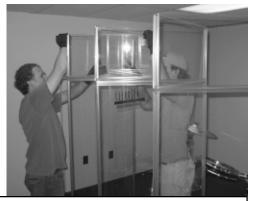
6. Note hinge configuration of large shield system. Be sure AX will be able to fold 180 degrees in same direction as the base system once installed. Use your ladder if needed and have your assistant "feed" the folded AX panels one at a time while you place them into position atop the larger shields. Make sure edges line up. Don't seat AX panels completely until all are in place. Tap top of AX panels with rubber mallet to seat completely into H-channel.
