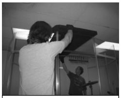
Lay rectangular STC on top center of IsoPac with at least a one inch over-hang in front and resting on support bar in back.
